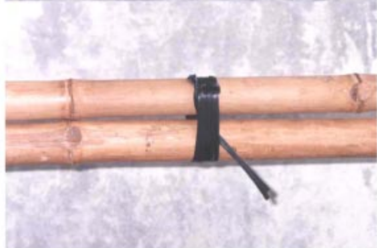
Figure 6.2 Tightening sequence of a lap in parallel members (continued)
