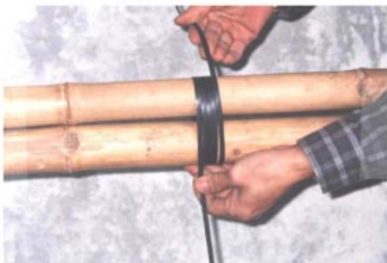
Figure 6.2 Tightening sequence of a lap in parallel members
