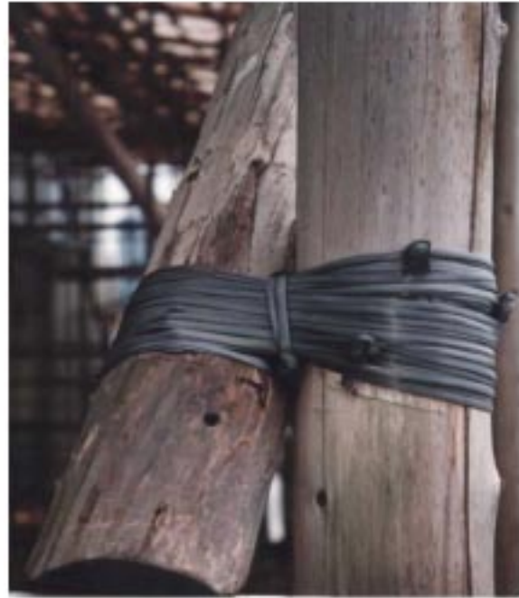
Figure 6.1 Knots in bamboo scaffolds (continued)
