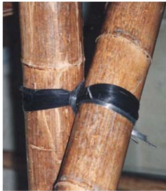
Figure 6.1 Knots in bamboo scaffolds
